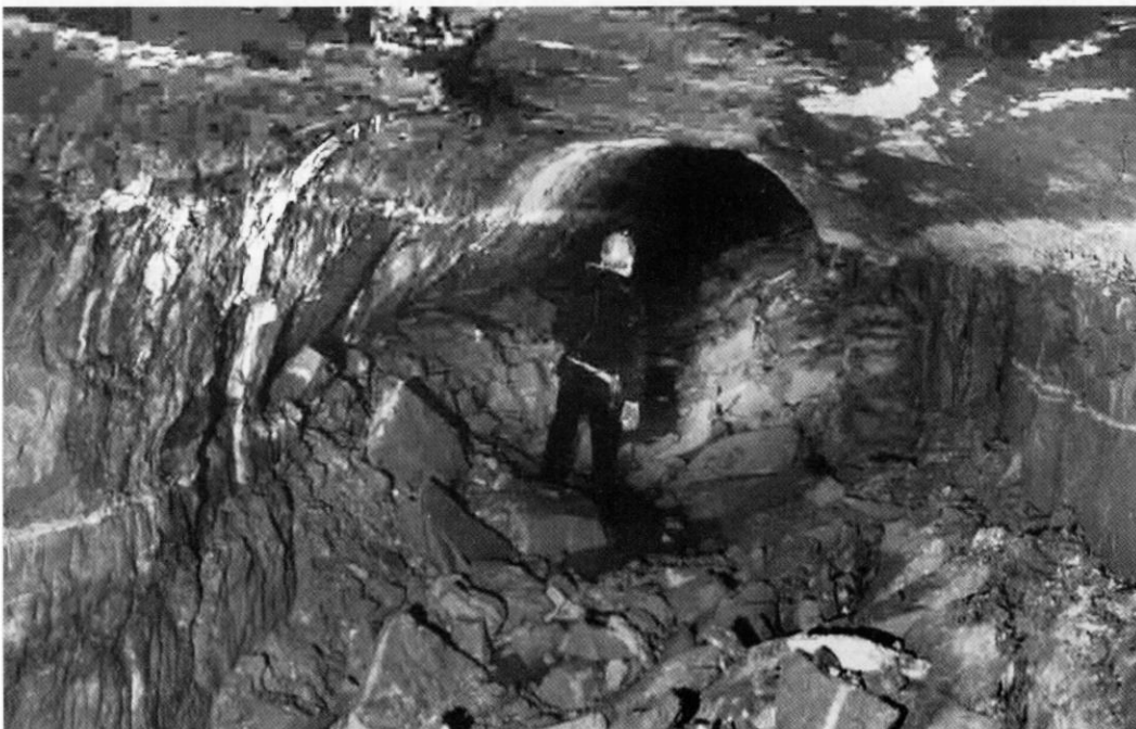
Inside the railway tunnel. Photo Peter Glanvill
